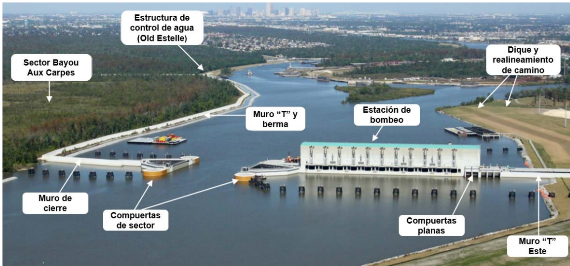
Figura 3-1. West Closure Complex, New Orleans, USA (US Army Corps of Engineers, 2021)
