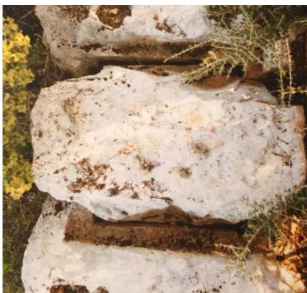
Figure 15. Repair of stone conduit, inserted stone element in situ , view from above. Note rectangular cuttings of the two neighboring guiding conduit elements (photo author).
