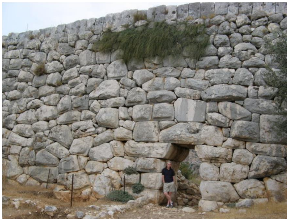
Figure 10. West view of cyclopean wall, stone conduit on top, the flat ashlar above the passageway carries the inscription. A similar passageway further to the left also shows an inscription above it, on the east side of the wall (photo by author).
