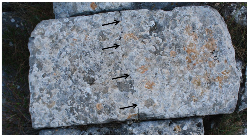
Figure 14. In situ conduit stone (90×90×50cm) of the Patara siphon, top view, with crack parallel to conduit axis (photo author).
