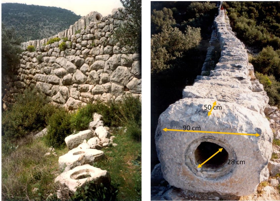
Figure 9. Left: the stone Delikkemer siphon of the Patara aqueduct on top of a cyclopean wall; right: upstream side of the in situ stone conduit (photos author).
