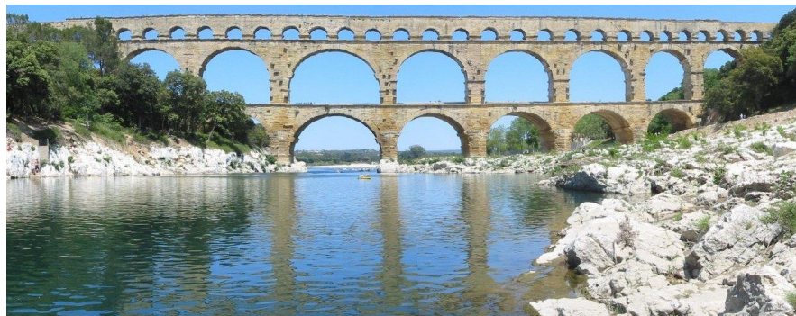
Figure 2. The Pont du Gard, 275 m long, and almost 50 m high (nl.wikipedia.org-wiki-Pont_du_Gard, March 2022).
