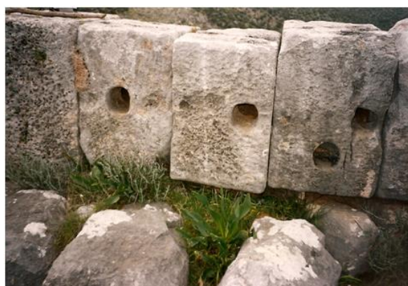
Figure 19. Deepest point of the Patara siphon, side view of stone conduit, with three holes to the bore to empty the siphon. The lowest hole does not connect to the bore (photo author).
