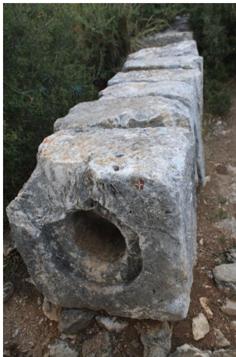
Figure 13. Final downstream conduit stone of the 182 in situ elements, with female joint (photo author).
